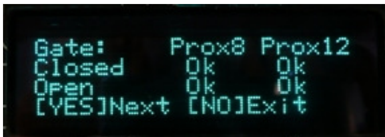
Figure 13 - Test completed and passed
