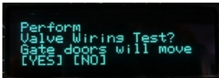
Figure 8 - Valve wiring test menu
