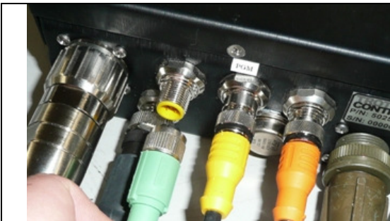
Figure 1 - Gate Angle Calibration Point
